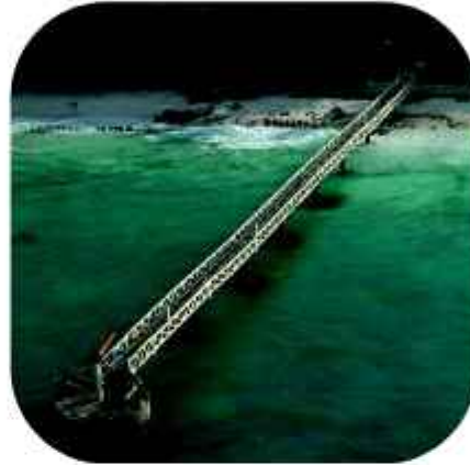
Low-Temperature Thermal Desalination plant at Kavaratti island, Lakshadweep
