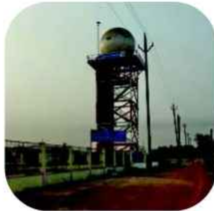
Doppler Weather Radar at Raipur, Chattisgarh
