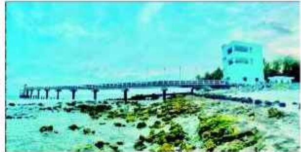
Fig. 2.1.9 LTTD plant at Chetlat Island, UT Lakshadweep.
