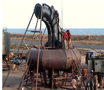
Buoyancy chamber being assembled to the main elbow
