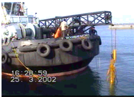
Use of Truss with tug (without a crane)
