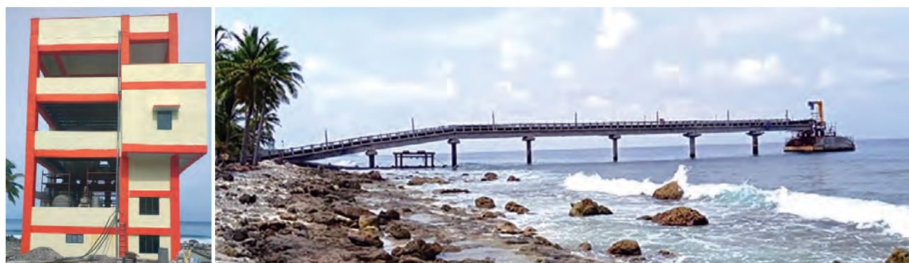
Fig. 3.14 Views of the Sump, Trestle and Plant building of Kalpeni LTTD Plant
