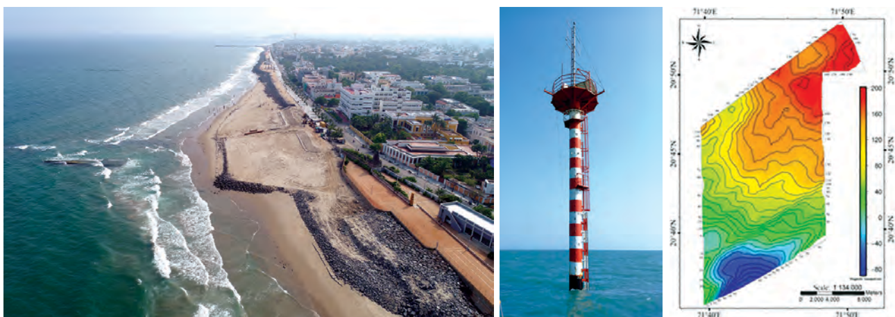
Fig. 3.15 (a) Performance of the Submerged Reef (b) Installed LiDAR based Data Collection Platform, and Geophysical investigation at Gujarat.
