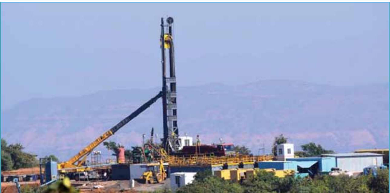
Fig. 5.4: Snapshot of drilling rig at Pilot borehole site
