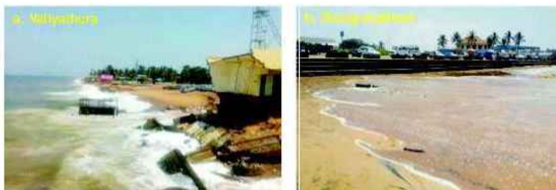
Fig.5.31: Field photographs of Valiyathura – Shangumukham stretch during the event on 18 March 2019.
