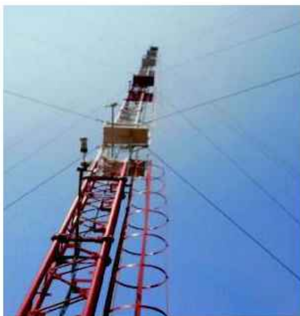
Fig. 2.3 Instrumented a 72-meter tower for measuring atmospheric GHG and other meteorological variables at ART facility.
